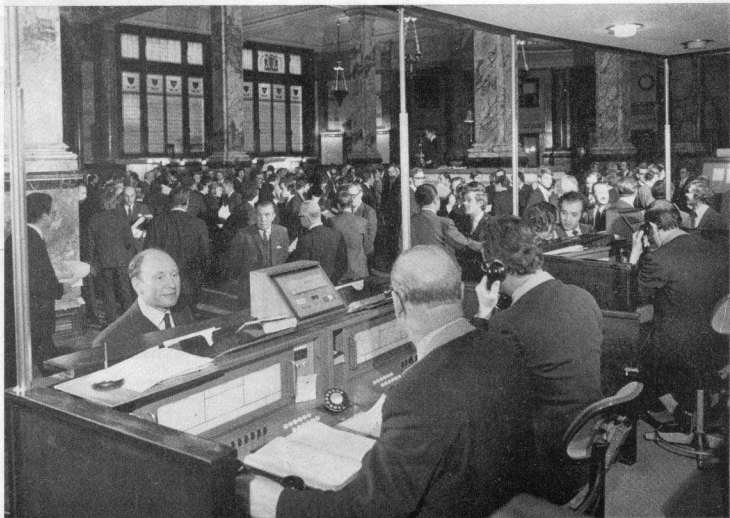
A general view of the floor of the Baltic Exchange with the telephone switchboard in the foreground.
